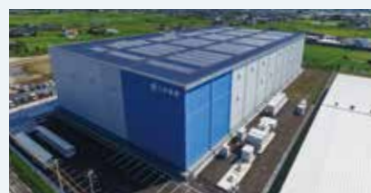
The Mitsui-Soko's Kanto P&M Center, where fluorescent lighting panels and LED lighting were installed.
