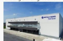
■ Construction Image Kanto P&M Center Existing Buildings A Exterior
