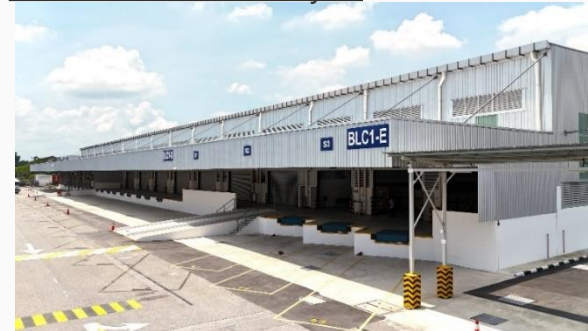
■ Warehouse in Malaysia
